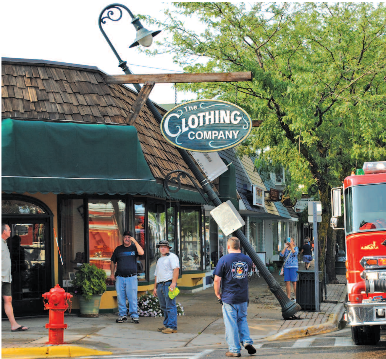
A lamp post blew over in downtown Charlevoix recently as a result of the quick wind and rain storm that blew through the area. The lamp post landed on the Clothing Company roof. Fortunately the only damage to the building was to a couple of the wood shingles. The City of Charlevoix Fire Department responded very quickly.
